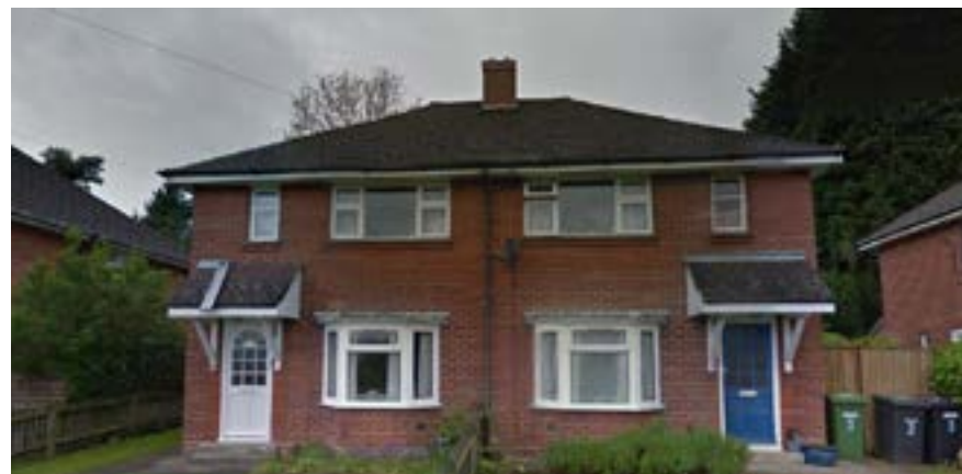
3-4 Peewit Hill – 2 storey semi-detached 80s style houses
