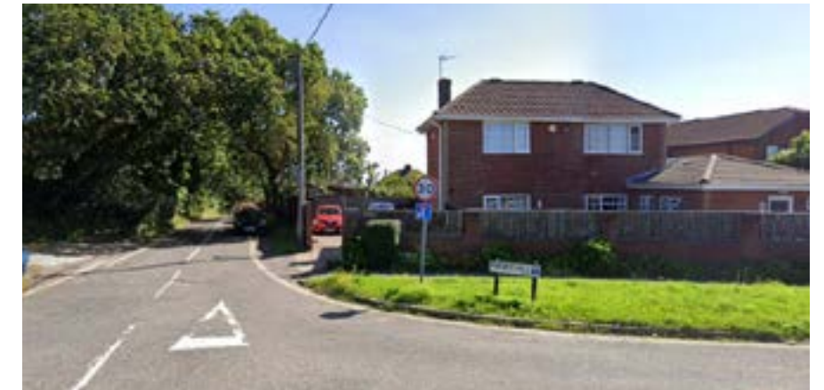
Entrance of Peewit Hill – 2 Storey Care Home
