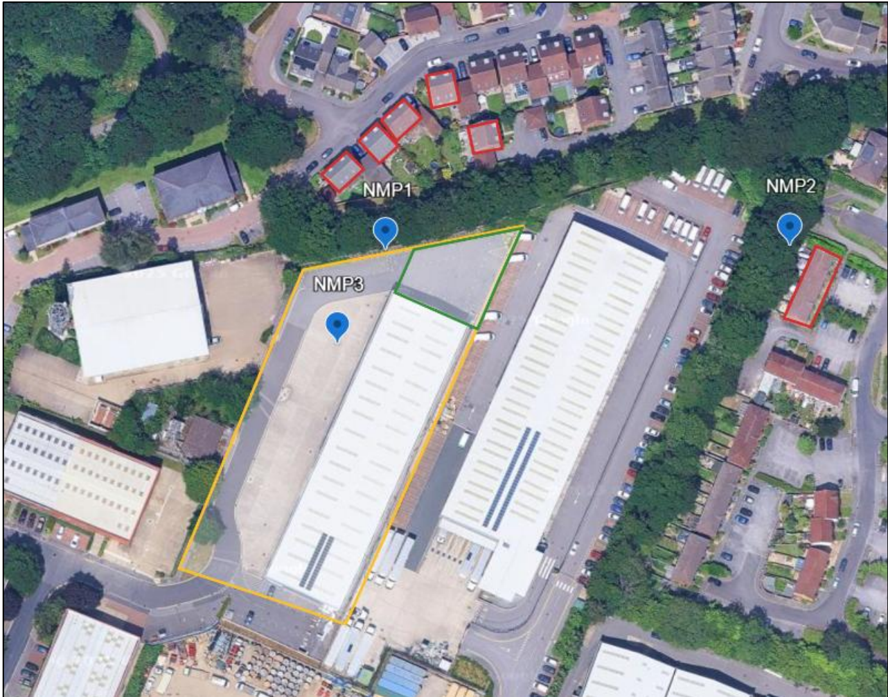
Figure 2: Site Location and Noise Measurement Positions
