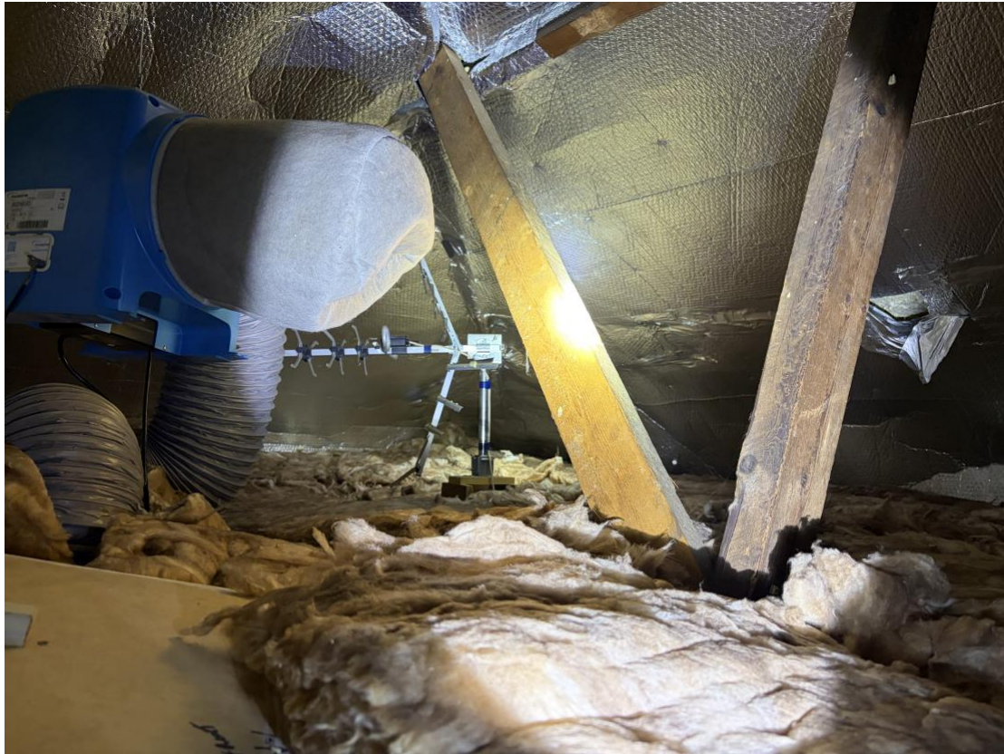
Figure 6. Loft space of 57 Woolston Road (May, 2026).
