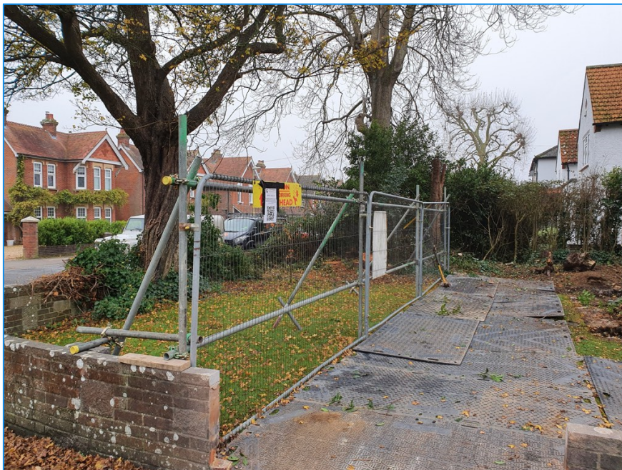
Tree protection barriers & trackmat ground protection
