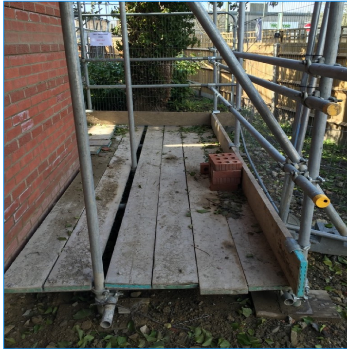
Tree protection barriers and scaffold ground protection
