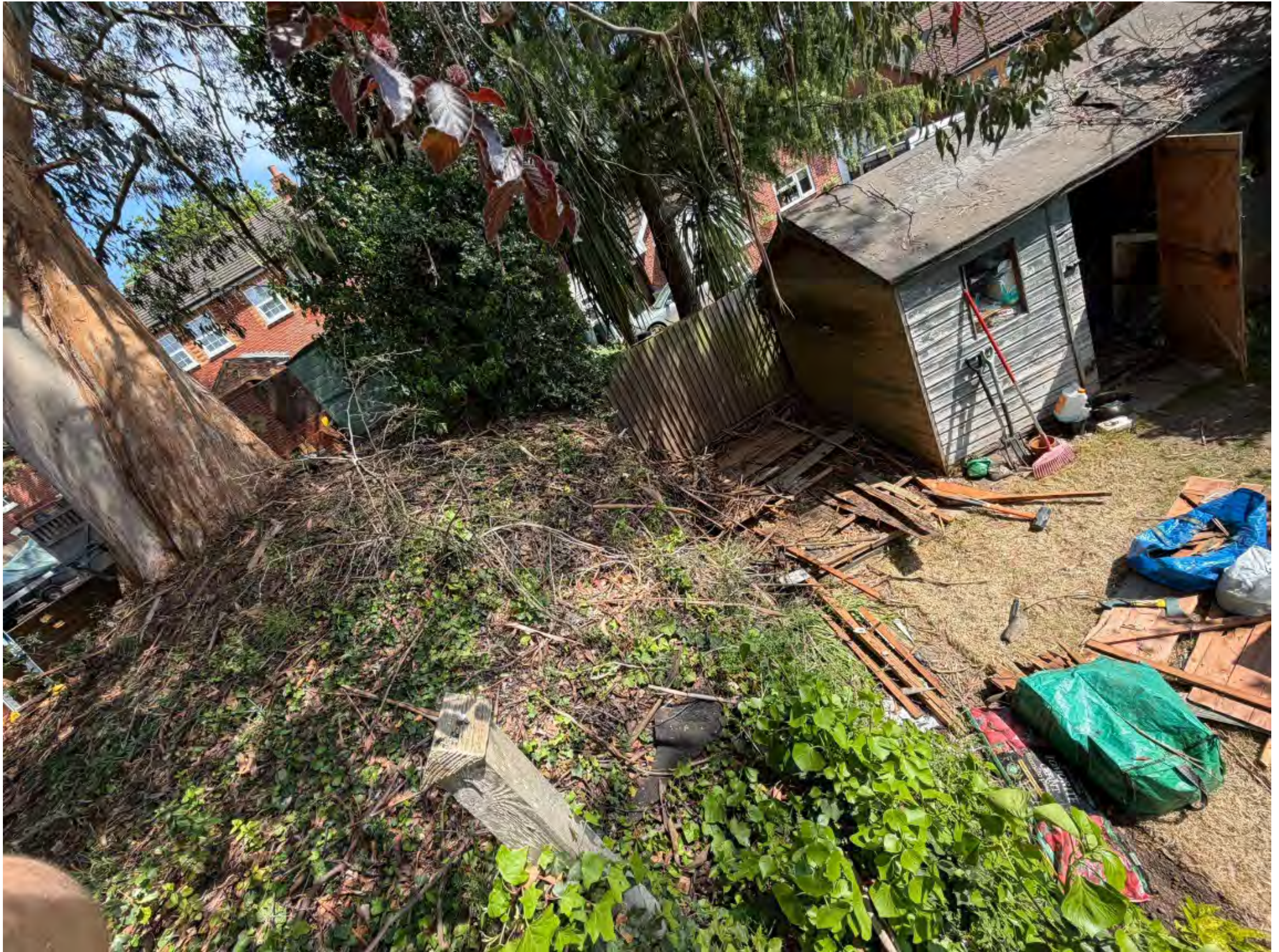
Image 9: View from within the subject property south-eastward, showing the approximate 3m step-down to the neighbouring property boundary. The retaining wall, which lies out of frame to the right, separates the two levels. The extent of the crown's southward spread over this level.
