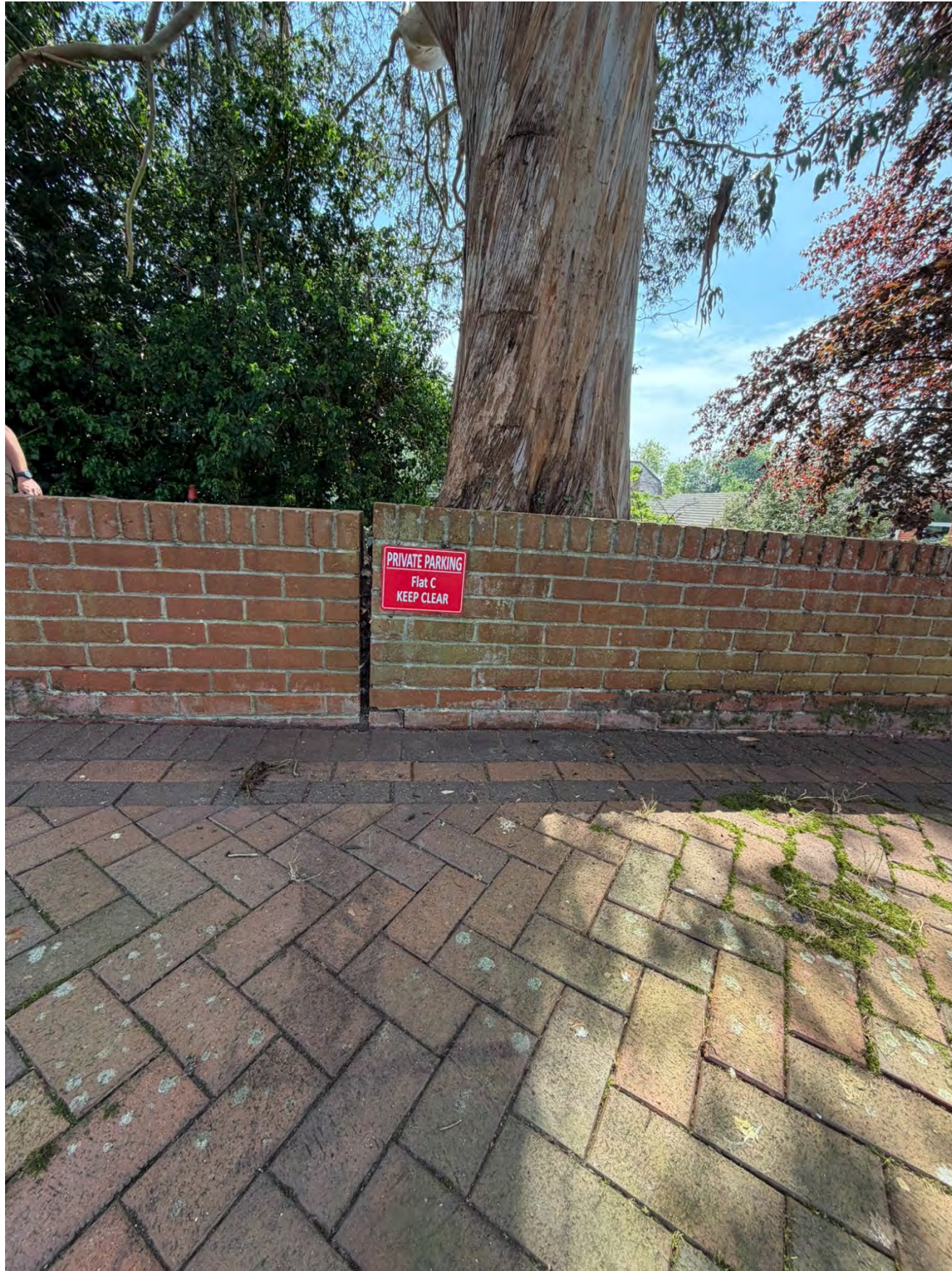
Image 5: Low brick wall separating carpark on NNW aspect showing vertical gap and displacement consistent with root-related ground movement. The subject Eucalyptus stem is visible in the background.
