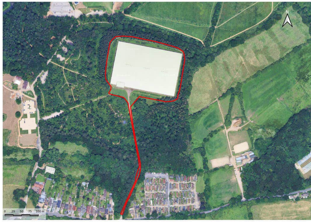
Figure 1. Site Boundary (Portsmouth Water)
