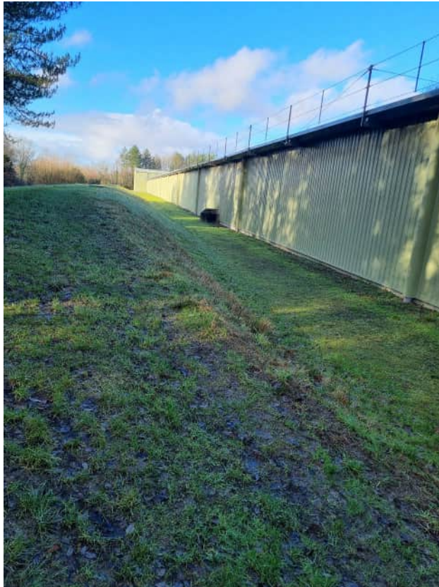
Figure 7. View of the building on-site (taken January 2026)
