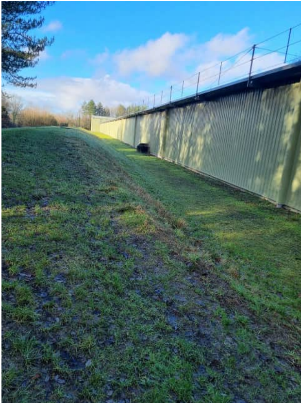
Figure 7. View of the building on-site (taken January 2026)
