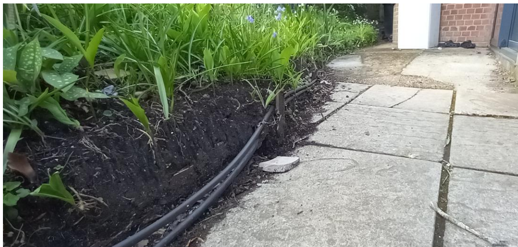
Photo 1 Low retaining wall removed to east of T1. The paving is the patio area in the drawing below
