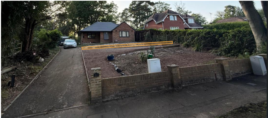
Photo 2 Location of retaining wall west of parking area. Viewed from road.
