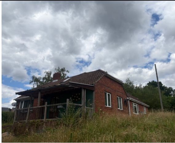
Photograph 7. The southern elevation and view of the garden.
