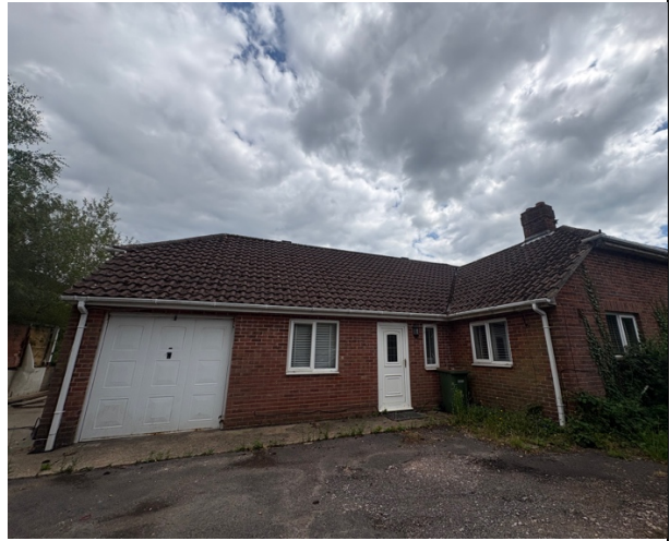
Photograph 2. A view of the western elevation and driveway.
