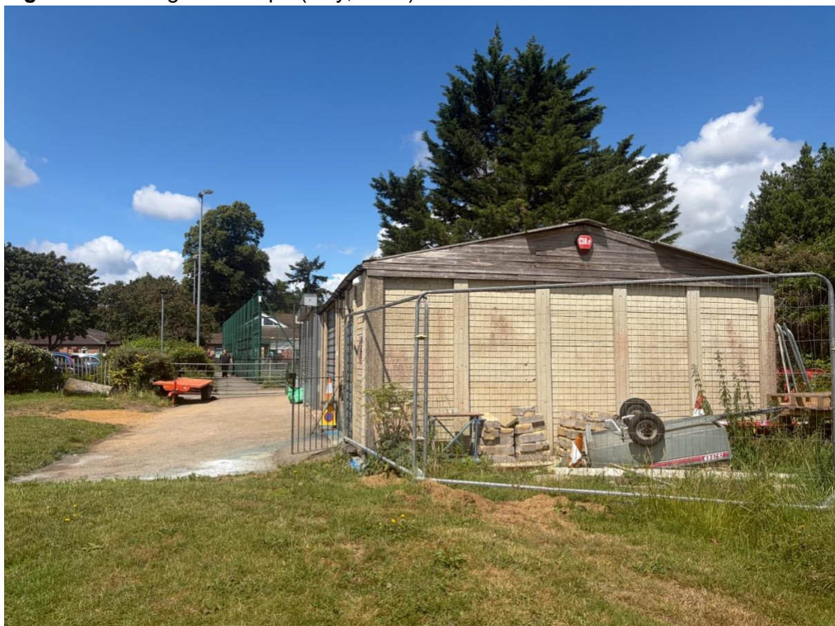
Figure 3. Existing workshope (July, 2026).
