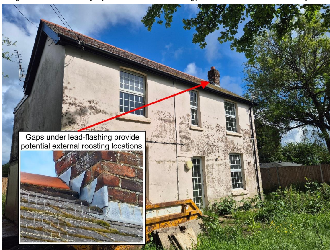
Image 4.3.1.1. Location of a potential external roosting feature on the south elevation of the house.
