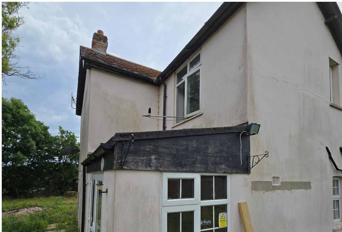
Photo 2 Location 2. Side façade facing Animal Welfare
