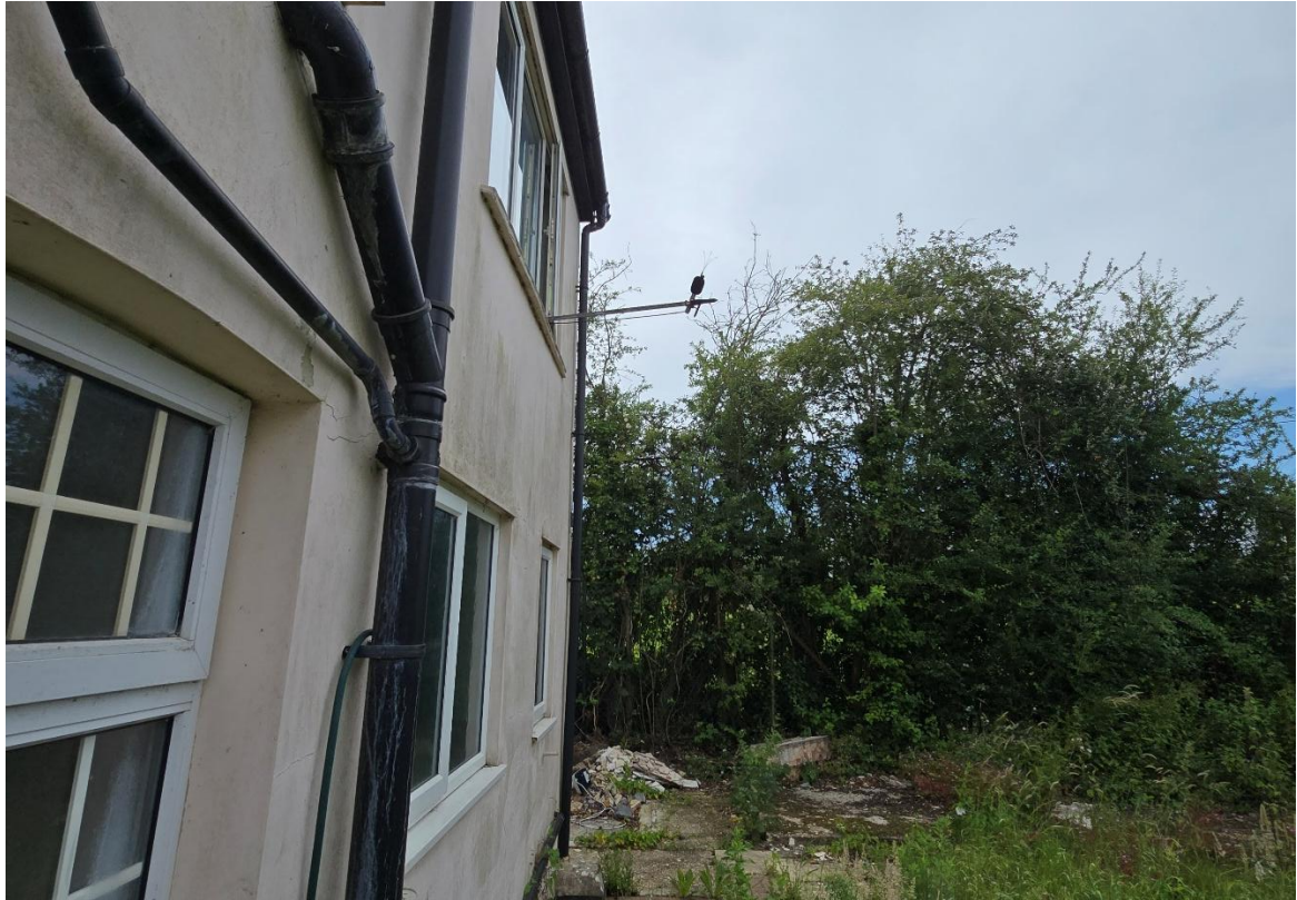
Photos 1 Location 1. Rear façade
