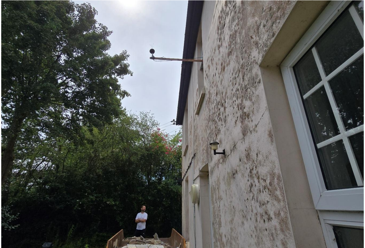
Photo 3 Location 3. Front façade facing Mortimers Lane
