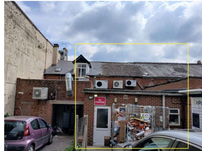
Western elevation of B1.
