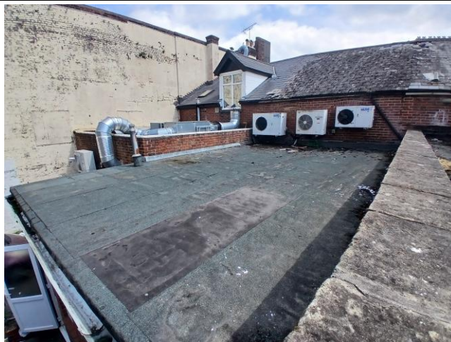
Photo 3: Western flat roof extension.
