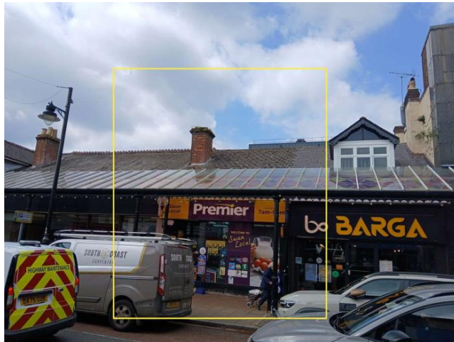
Photo 1: Eastern elevation of B1.
