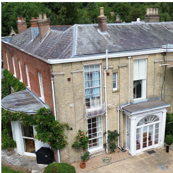
Front right hand corner of the main property showing the portico (taken by drone on 18.06.26)
