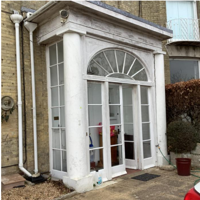
Photograph taken from the front left of the portico structure (photo taken 06.01.26).
