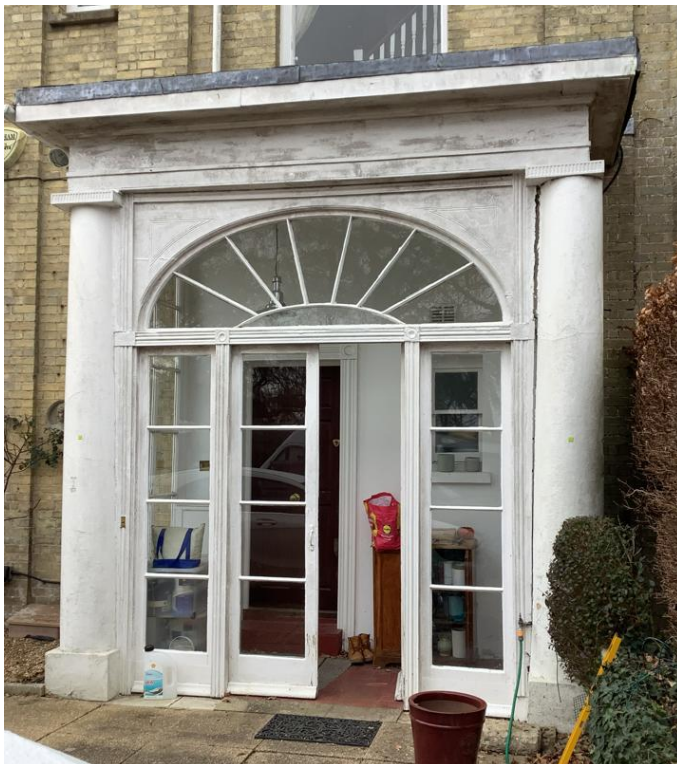
Photograph taken of front elevation of portico allowing for the 2 columns to be compared (taken 06.01.26)
