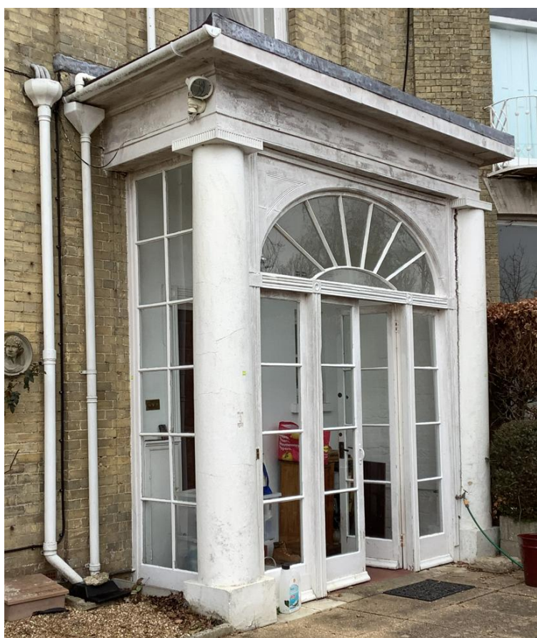
Figure 5: Photo showing the front portico in question
