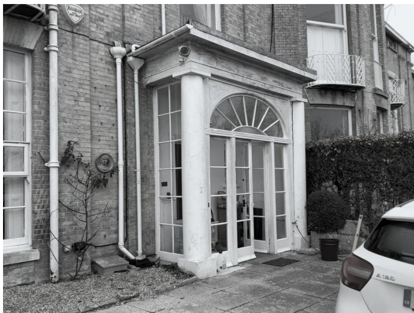
Figure 1 – view of area of works – front portico structure
