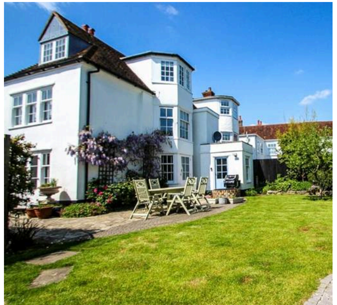
View of the garden area and existing dormer from the South-East
