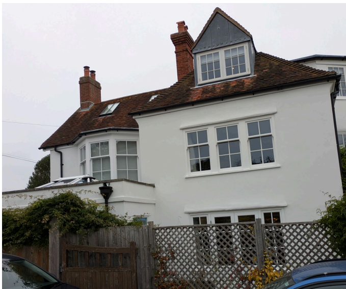
View of the south elevation and rooflights
