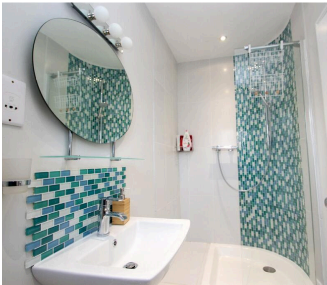
Modern existing ensuite finishes to be replaced
