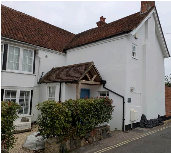
Street-level view of South House from the North-West
