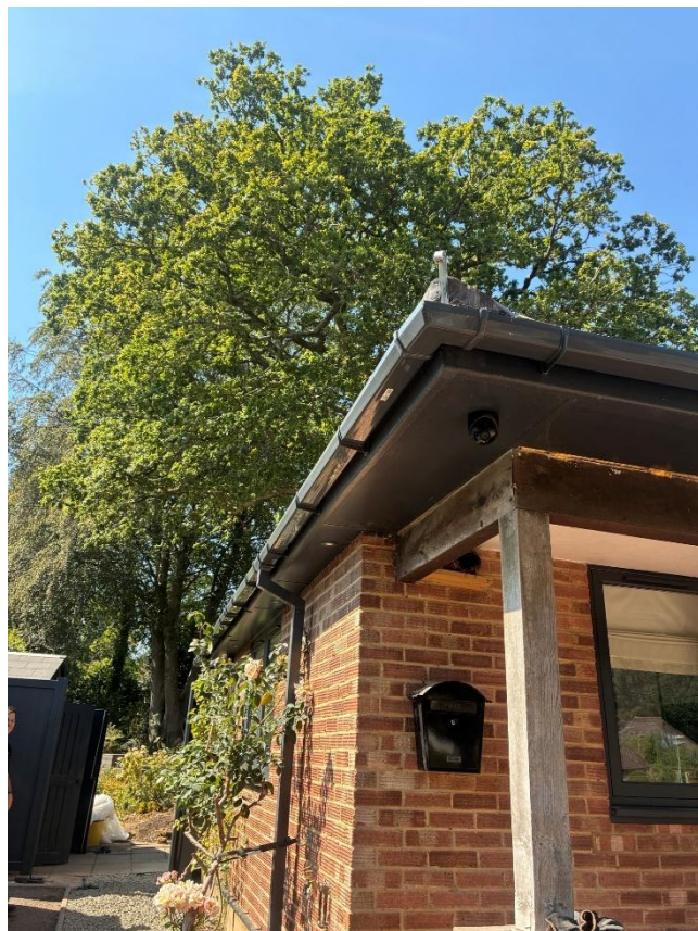
T2 Overhang over the extension
