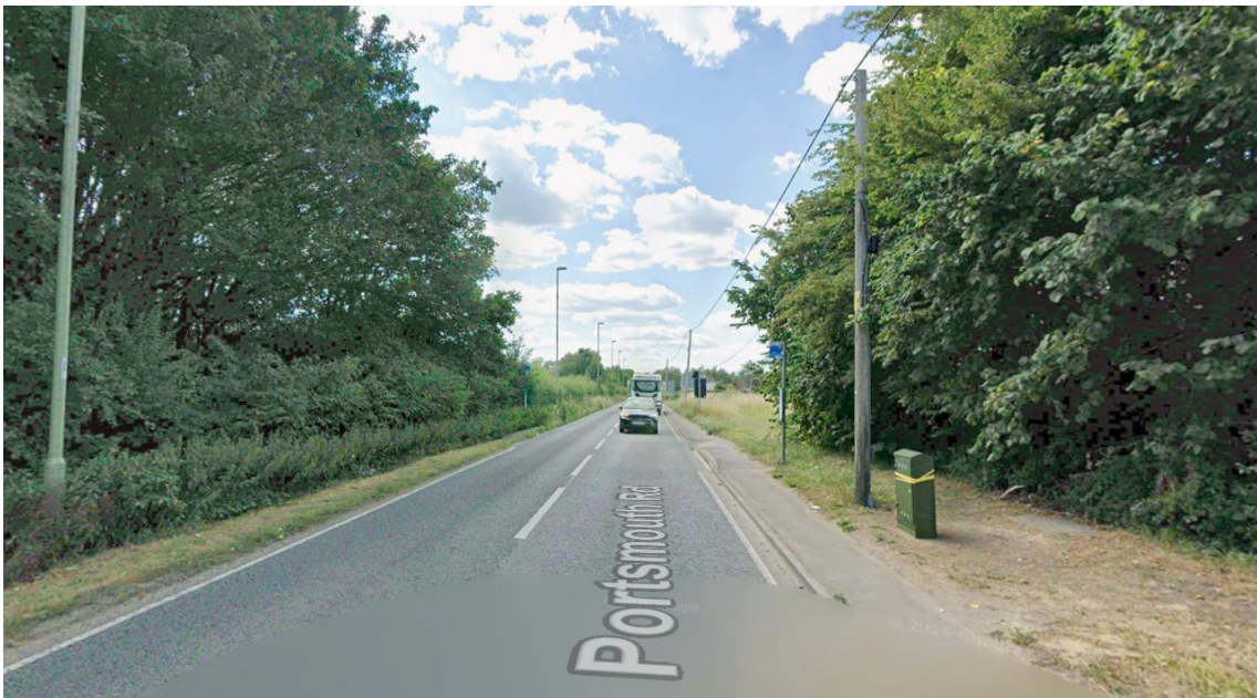
Bus stops, pavement and streetlights along Portsmouth Road (outside the site) – looking west
