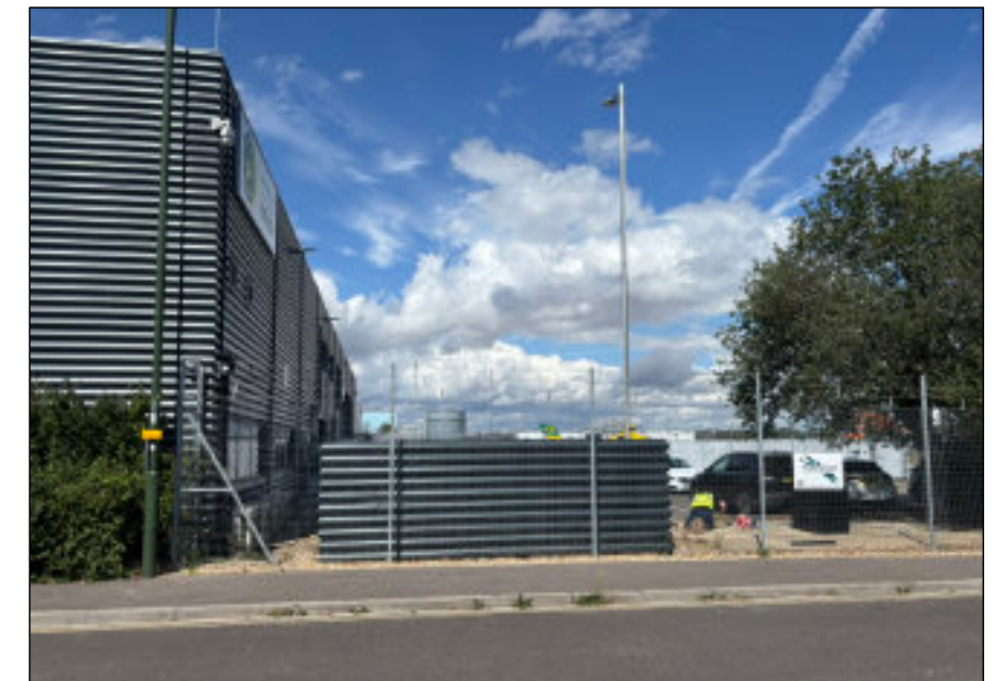
6. Existing Bin Store
