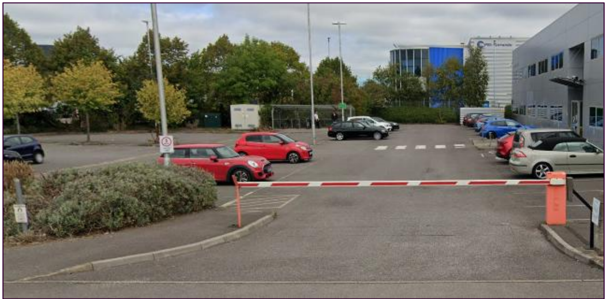
Image 2.1: Existing Site Access
