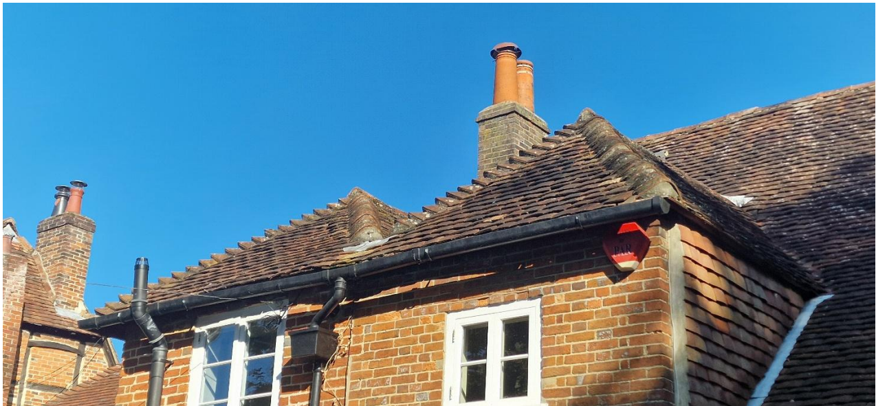
Picture 5: Showing the tile bed on the existing double-width dormer
