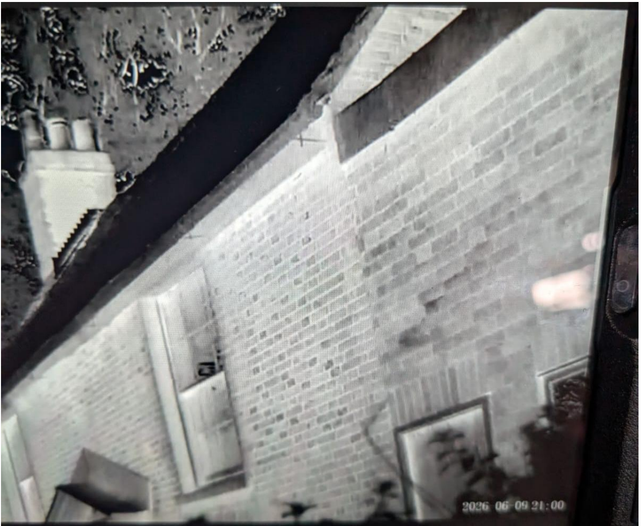
Picture 8: Showing the thermal of the front of the building
