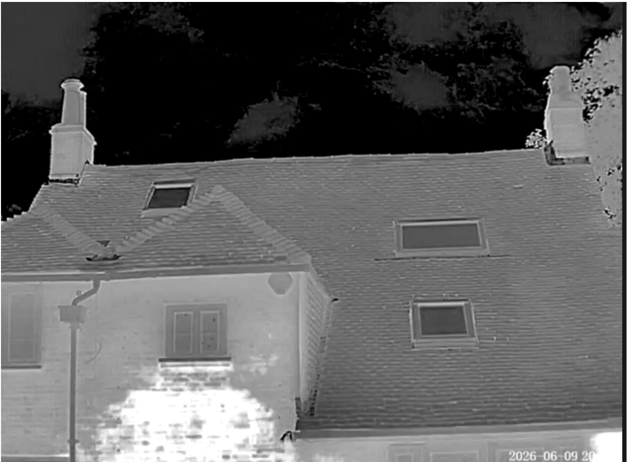
Picture 7: Showing the thermal image of the rear of the building
