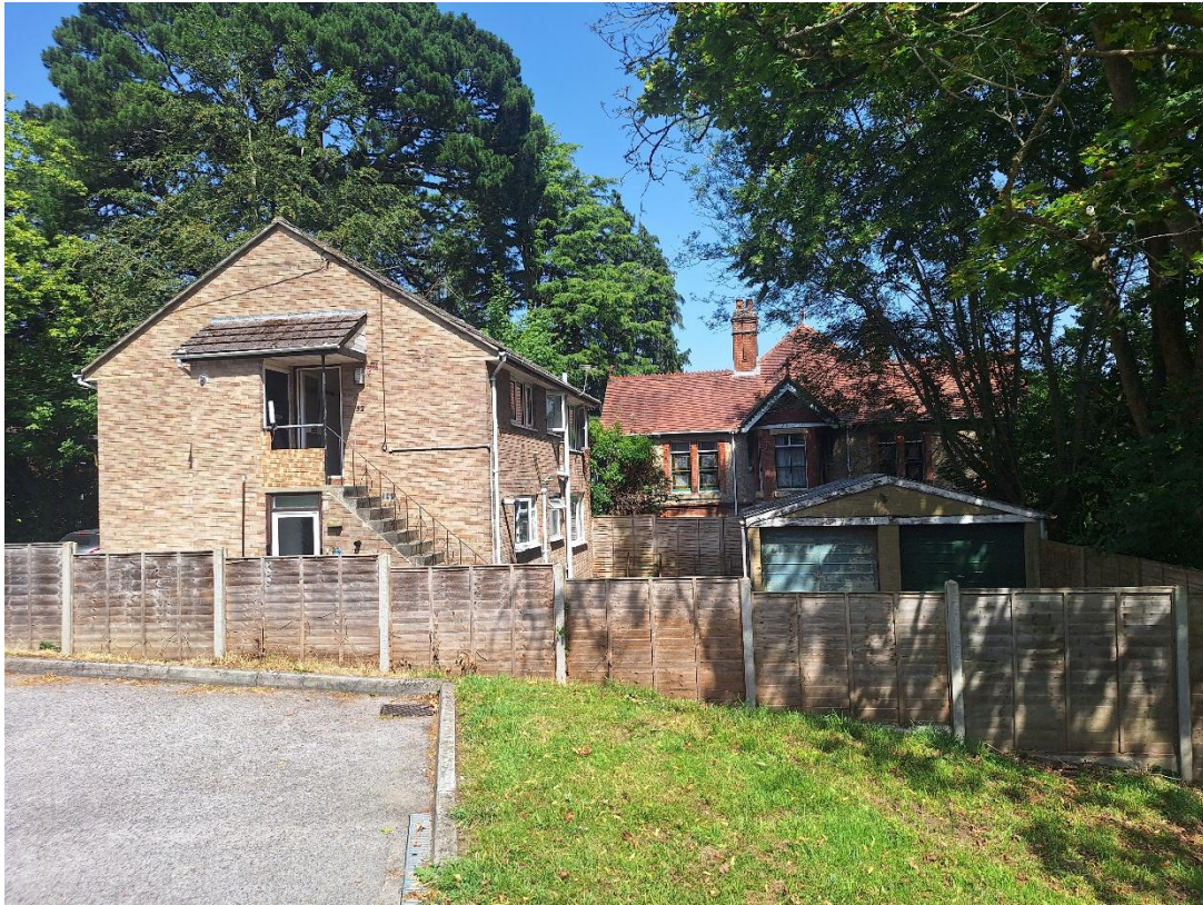
Rear Habitat showing garage
