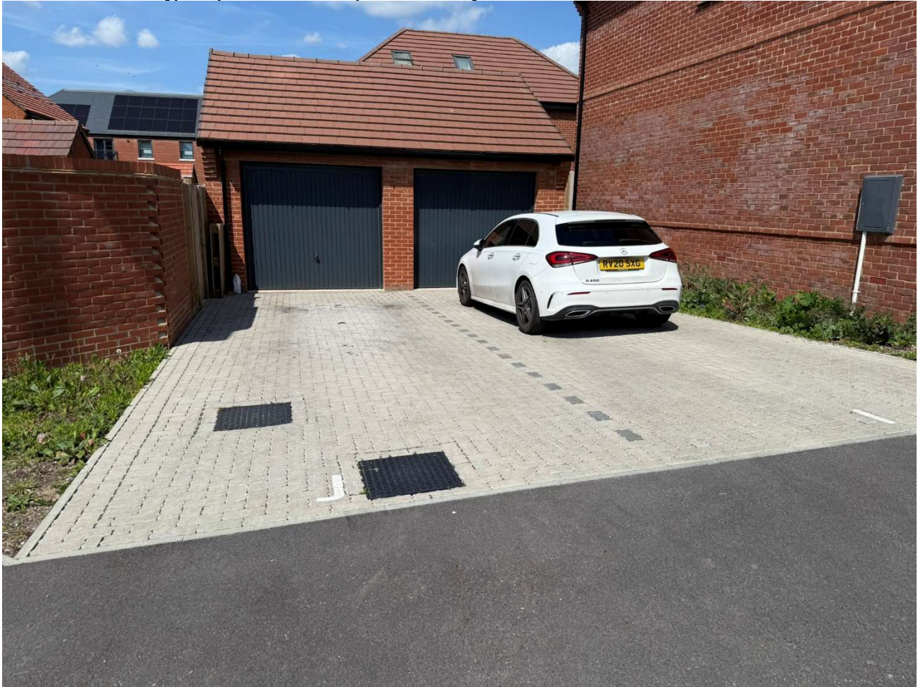
Photo 3: View onto typical permeable block paved driveway
