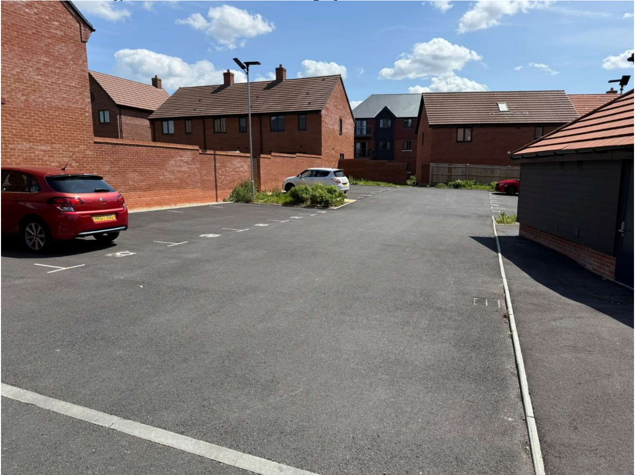
Photo 2: View onto typical macadam surfaced area with gully.
