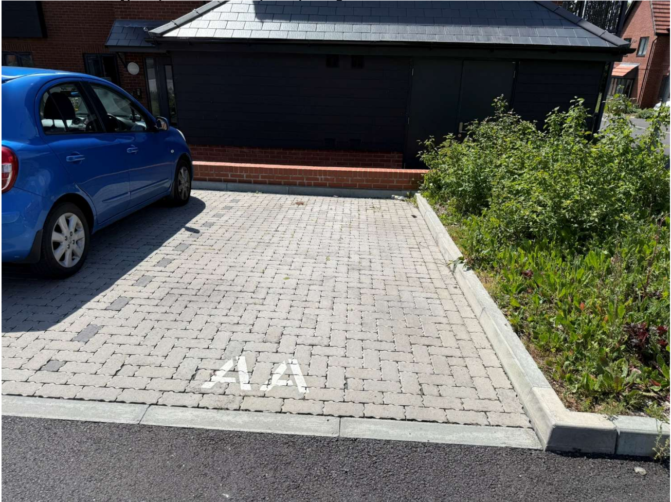
Photo 1: View onto typical permeable block paved parking area.
