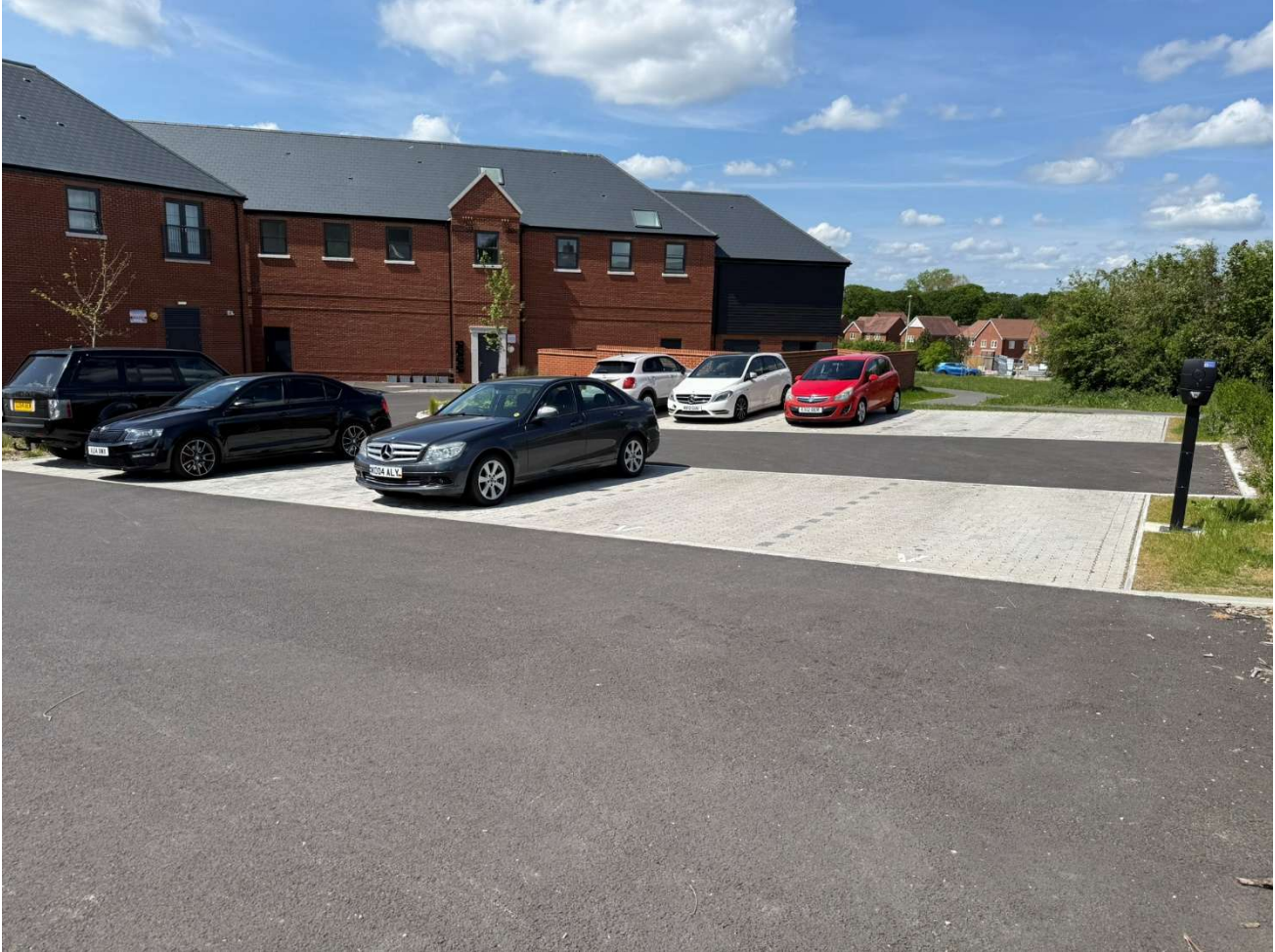
Photo 4: View onto typical macadam parking court and permeable block paving parking spaces.
