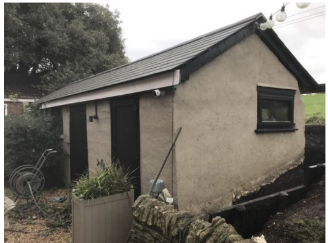
Image 10: Northern and western elevations of B2
