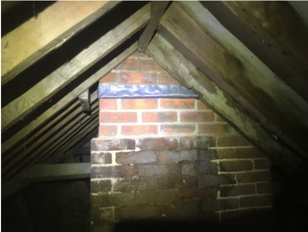
Image 23: Chimney in the centre in the northern area of the void
