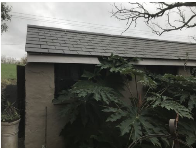
Image 11: Southern and western elevations of B2
