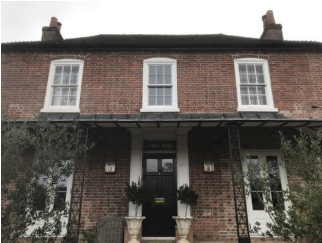
Image 12: Western elevation of B1, facing east
