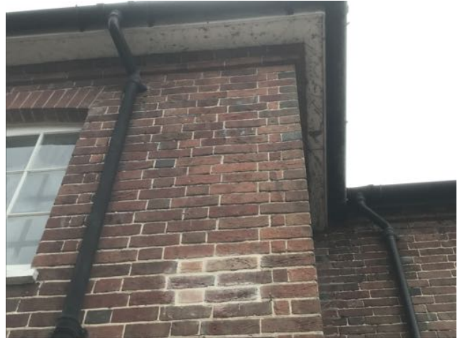
Image 18: Intact soffit box on northeastern elevation of B1
