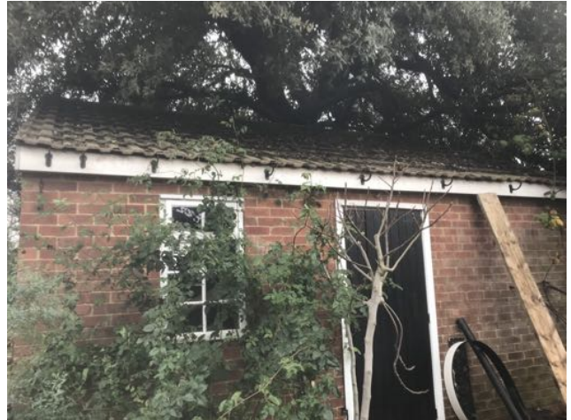
Image 8: Northern elevation of B3
