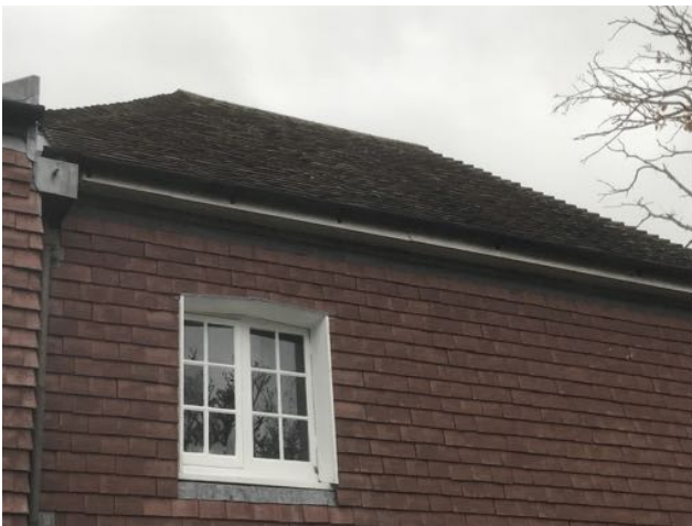
Image 19: Southern elevation of the roof of B1
