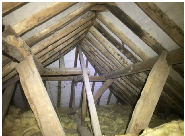
Image 22: Northeastern corner of the void
