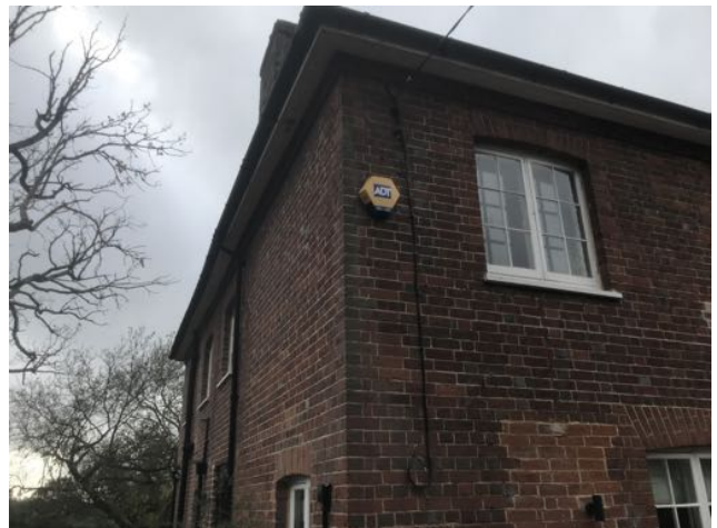
Image 15: Eastern elevation of B1, facing south
