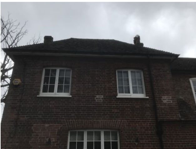
Image 14: Northern elevation of B1, facing south
