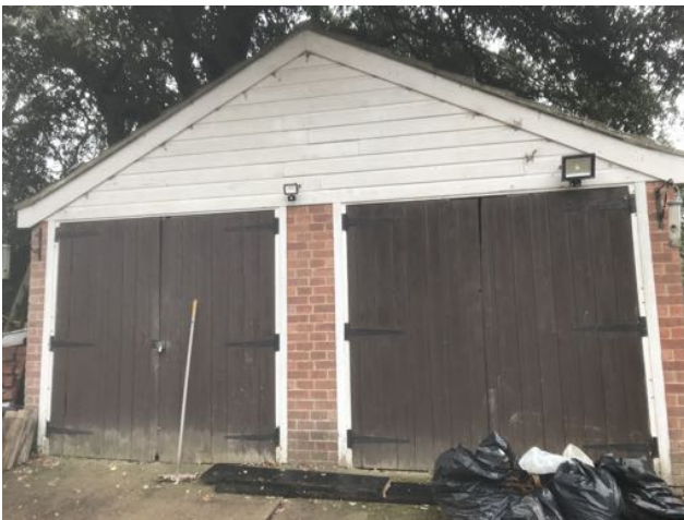
Image 9: Western elevation of B3
