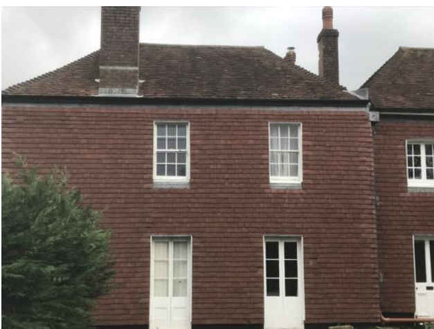
Image 15: Southwestern elevation of B1, facing north
