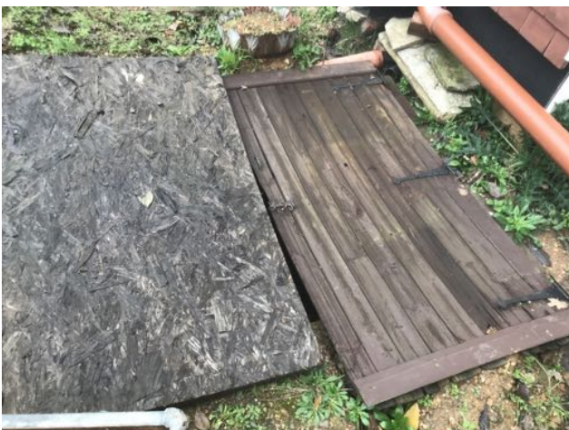
Image 27: External entrance to the cellar
