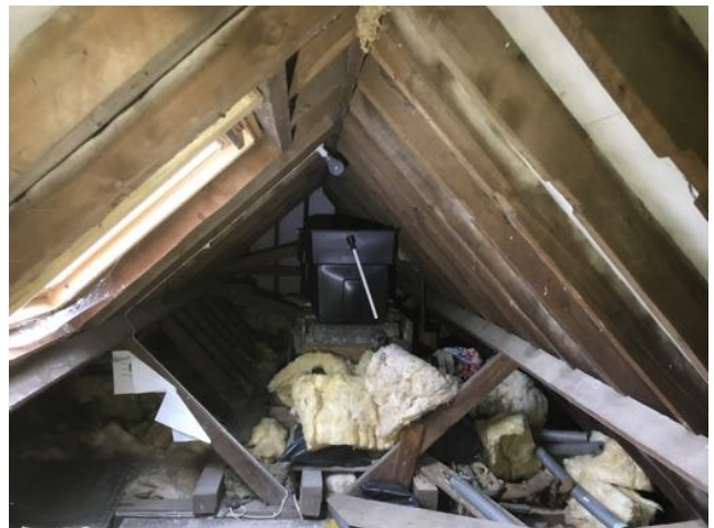
Image 20: Eastern area of the void, facing north
