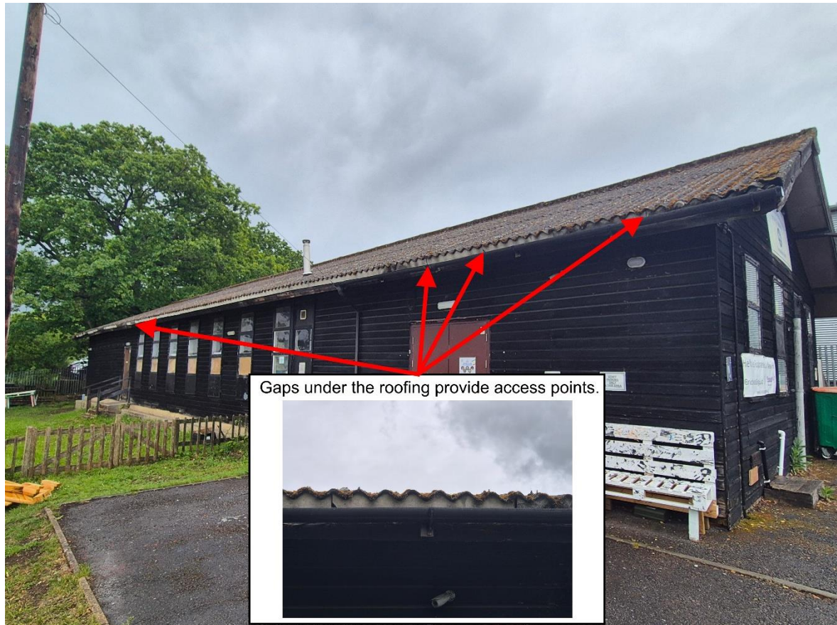
Image 4.3.1.4. Location of potential bat access points on the west elevation of the community building.
