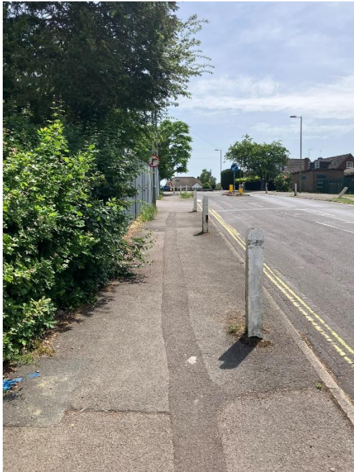
Photograph 2: Brickfield Lane pedestrian provision on northern side
