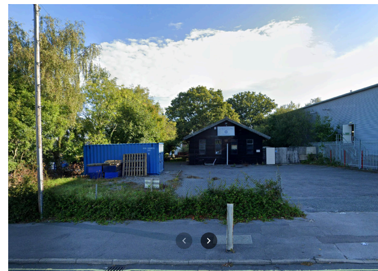
Current front elevation view from Brickfield Lane
