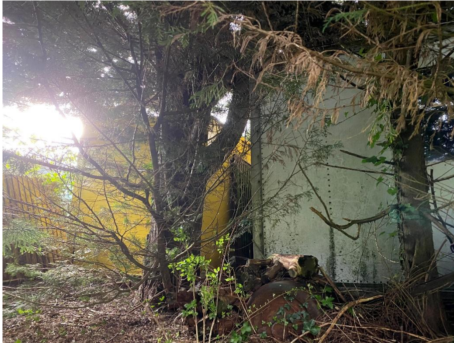
Figure 8. View of the buildings located within the hedgerow on site (taken April, 2024)
