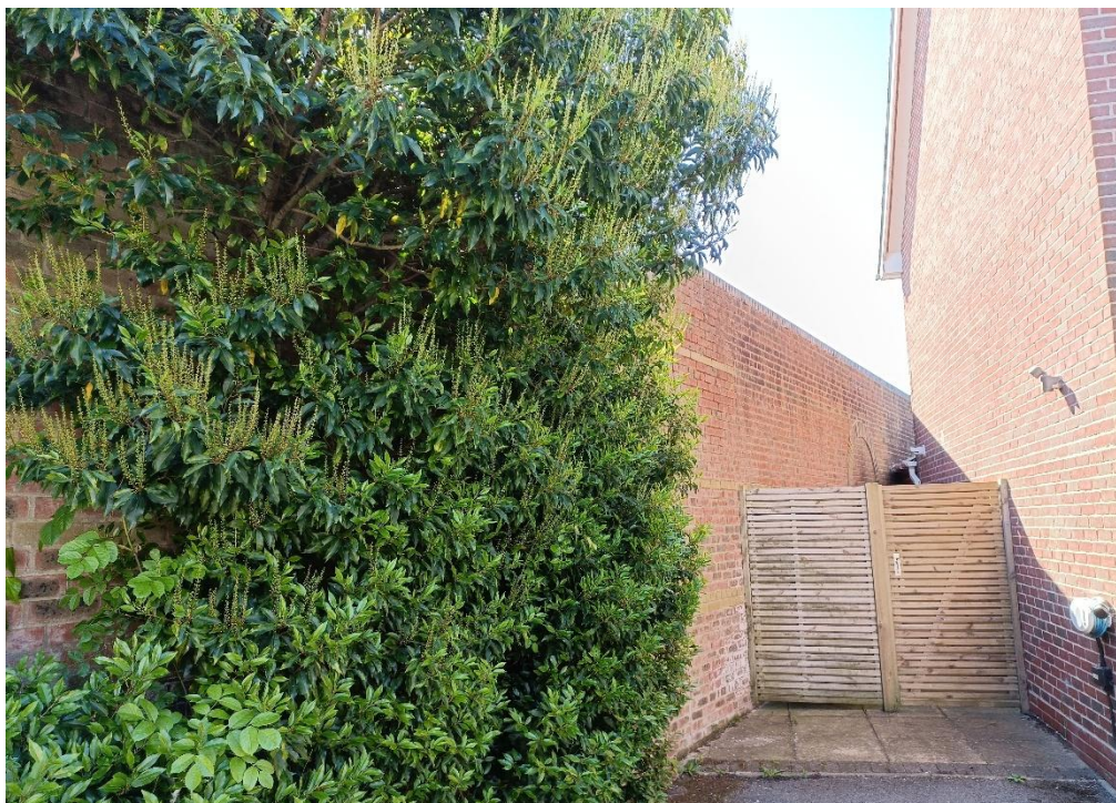
Image b): High boundary wall between Pitter Commercial Yard and dwellings at 12-20 Botley Road.
