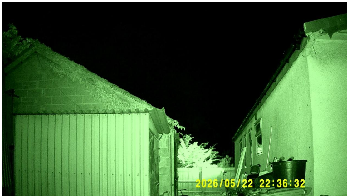
Figure 3.12: Screenshot of NVA Outputs at Darkest Point of Survey Buildings A & D (22/05/2026)
