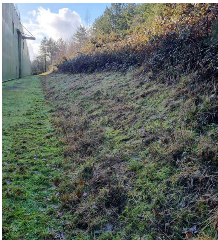
Figure 16. View of the bank to the north of the building (taken January 2026)
