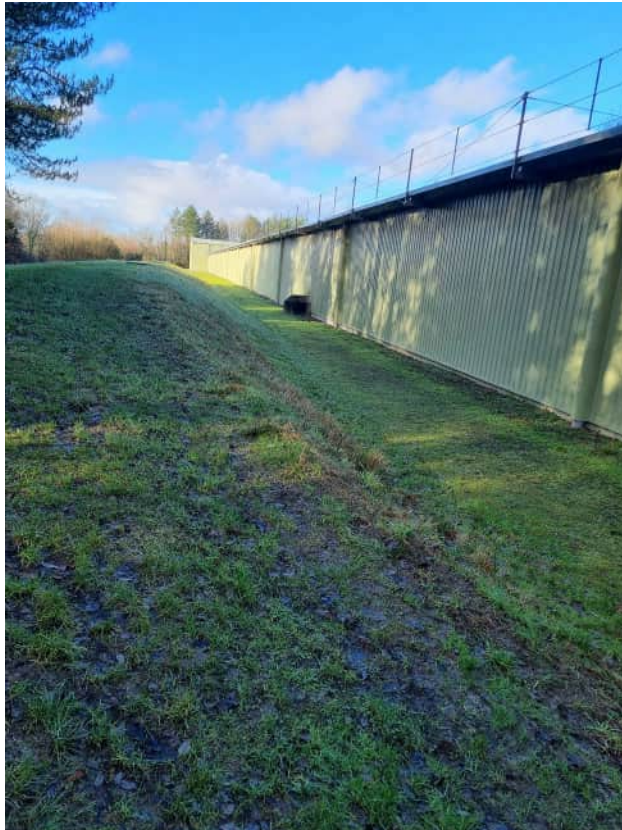
Figure 7. View of the building on-site (taken January 2026)
