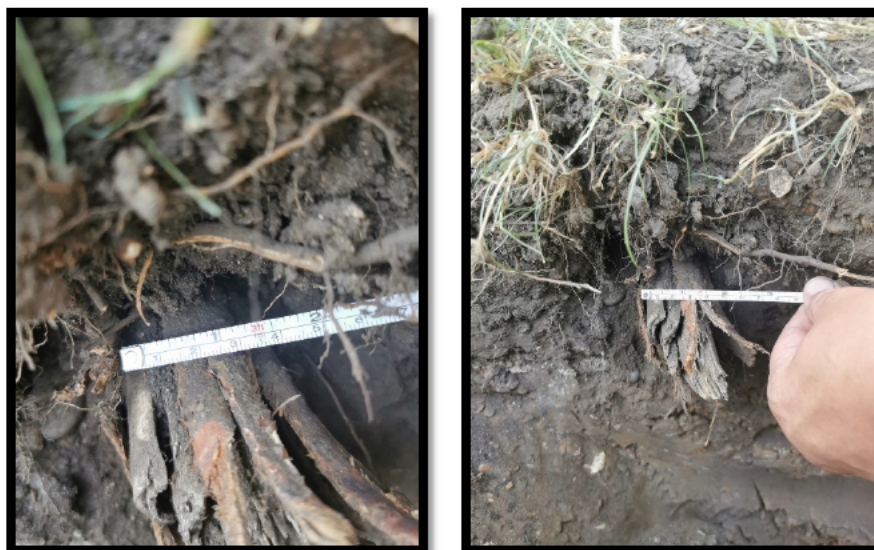
Plate 2 & 3: Tree root damage.
