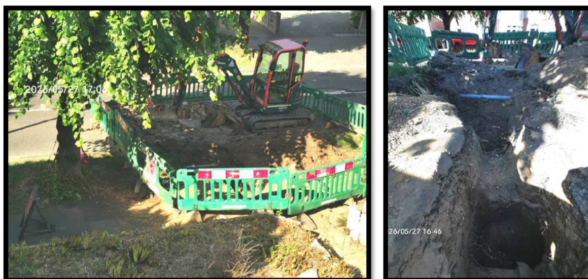
Plate 4 & 5: Extended trenching towards stem to locate pipework.
