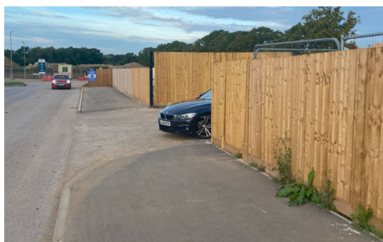
View west along Fieldfare Road with secure access to wheelwash beyond gate
