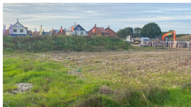
View of site looking south west with earth mound evident and wheelwash obscured behind
