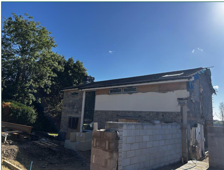
Photograph 2 – Main dwelling (B1), south-western aspect, showing the tightly bedded roof covering, sealed ridge and verge lines, and the eastern gable under construction with temporary sheeting.
