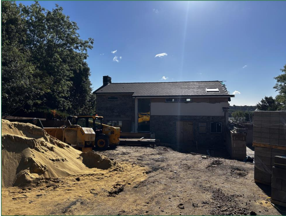
Photograph 7 – Wider site view showing compacted bare ground, stockpiled sand and aggregates, and plant on site.
