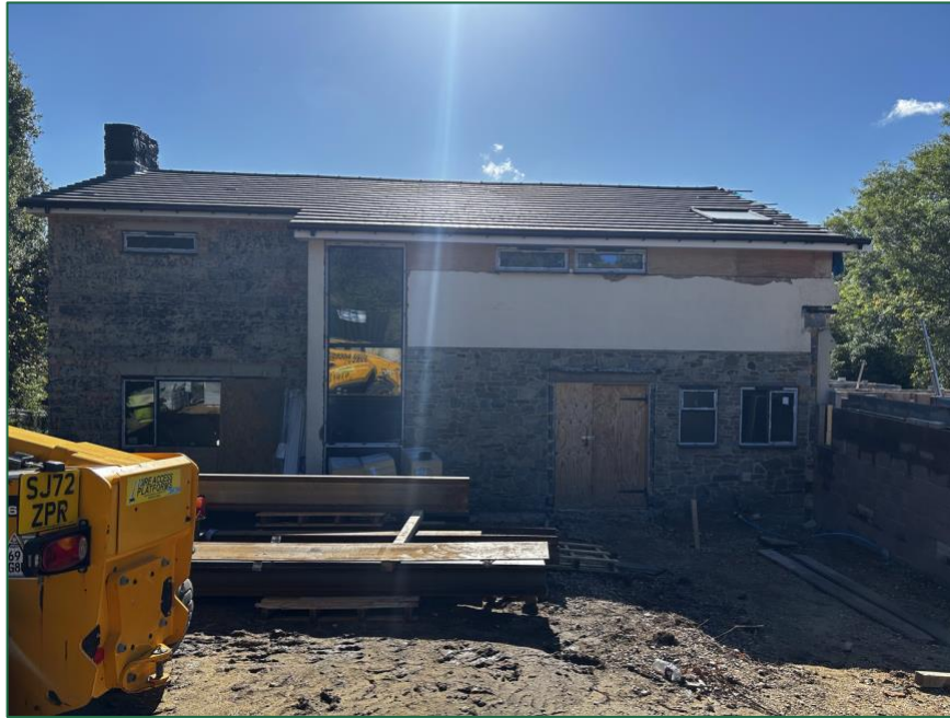
Photograph 2 – Main dwelling (B1), south-western aspect, showing the tightly bedded roof covering, sealed ridge and verge lines, and the eastern gable under construction with temporary sheeting.
