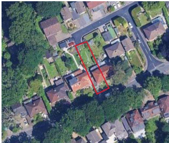
Aerial view of 91 Brownhill Road.
