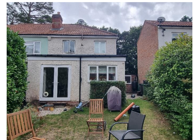
Rear façade facing North.
