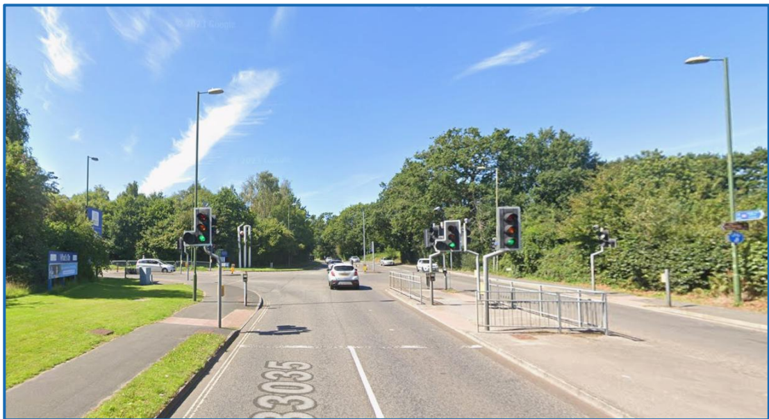
Figure 5: View of lighting layout on Botley Road at junction with Marshall Drive
