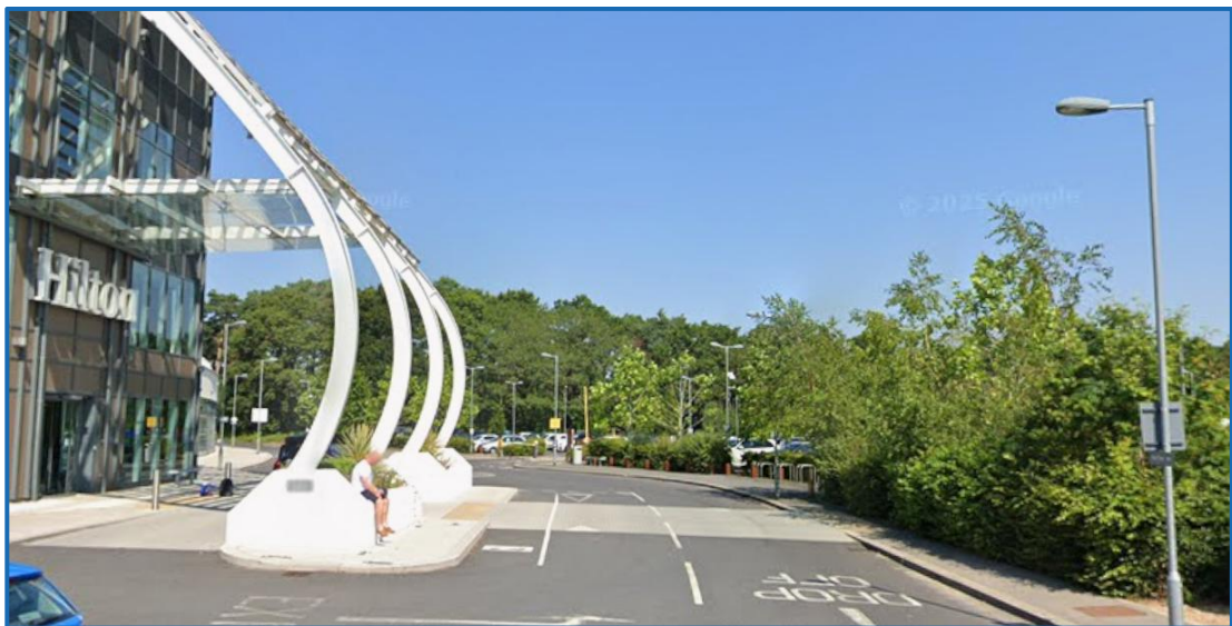
Figure 4: View of lighting at Hilton Hotel
