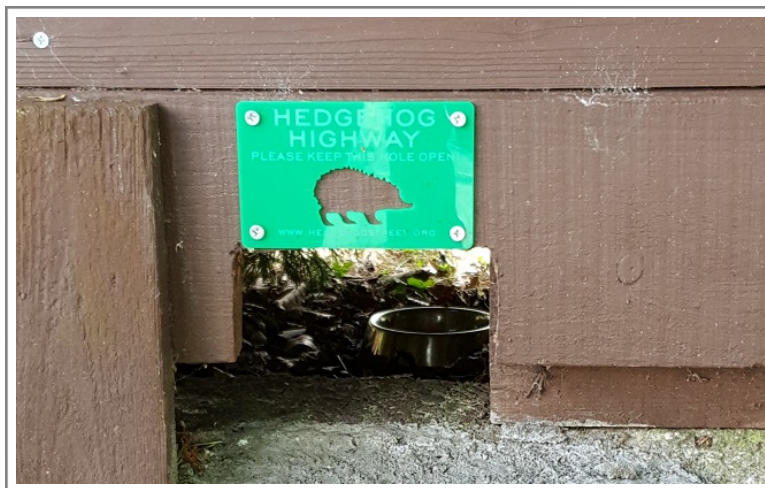
Example of a gap in the fence suitable for hedgehogs
