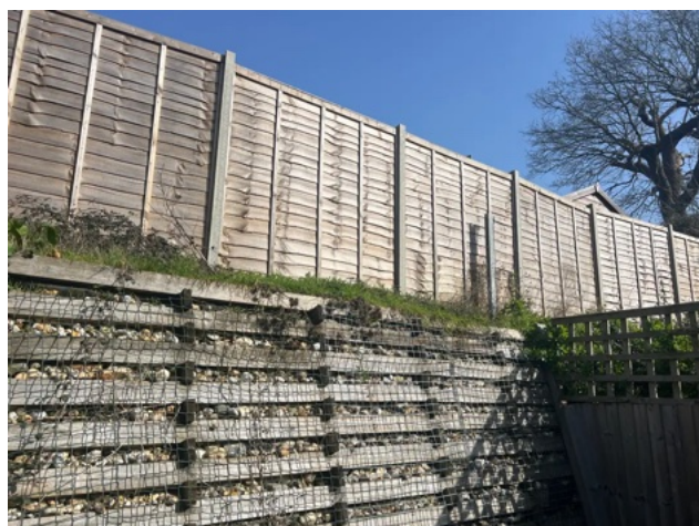
Image 2: The retaining wall, as viewed from the rear of no. 17.
