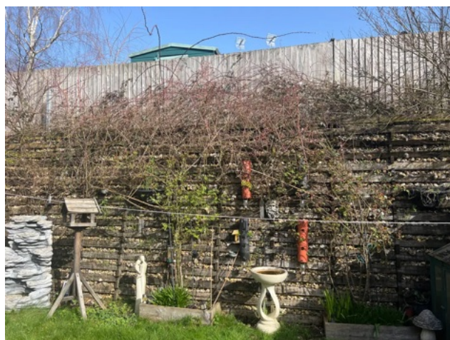
Image 6: The retaining wall, as viewed from the rear of no. 1.
