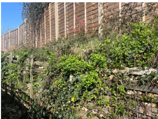
Image 1: The retaining wall, as viewed from the rear of no. 19.
