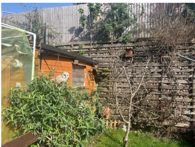
Image 5: The retaining wall, as viewed from the rear of no. 4.
