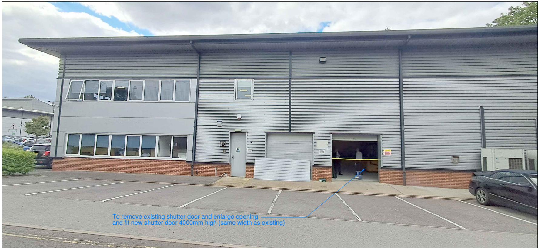
Existing West Elevation Photo
