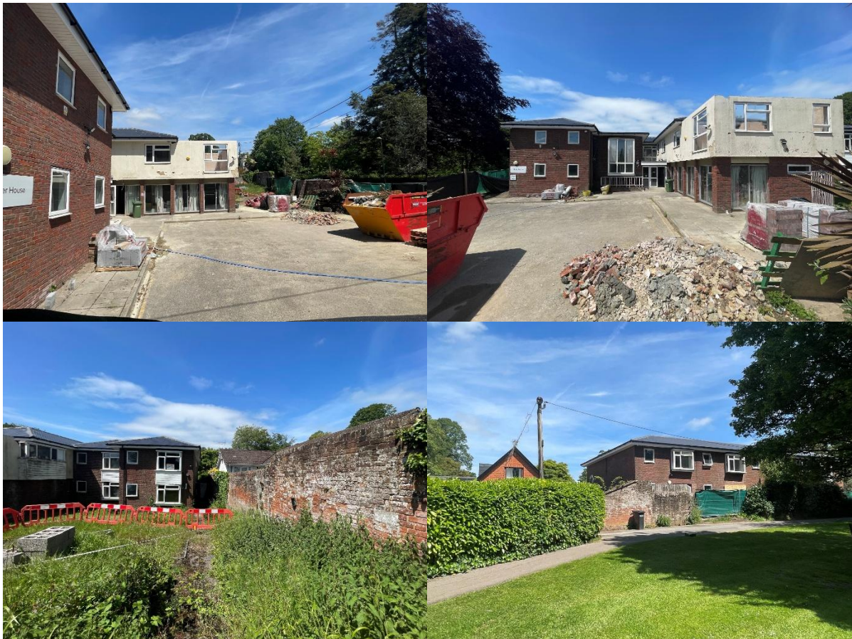
Figure 2: Photographs of the Existing Building
