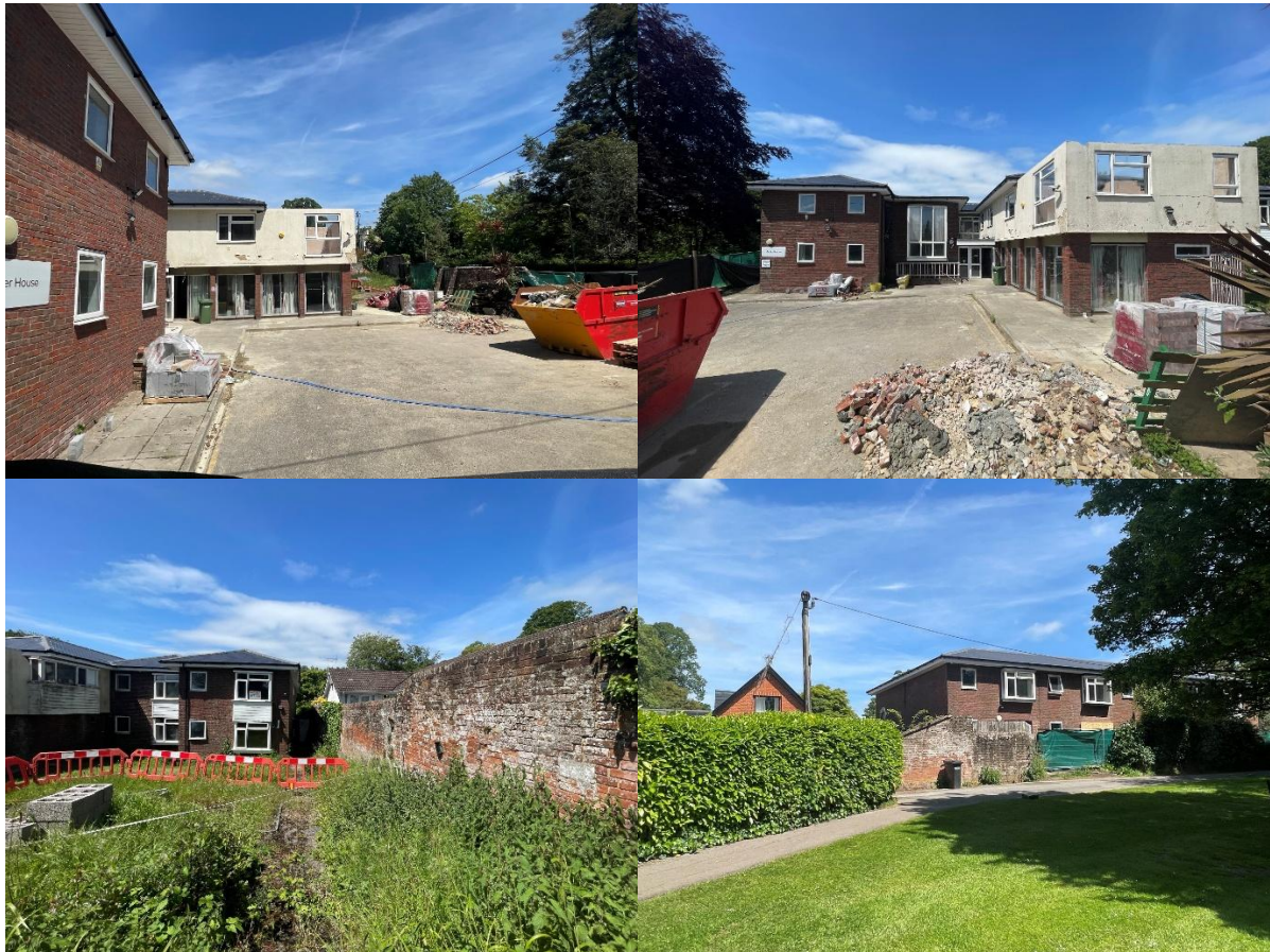
Figure 2: Photographs of the Existing Building
