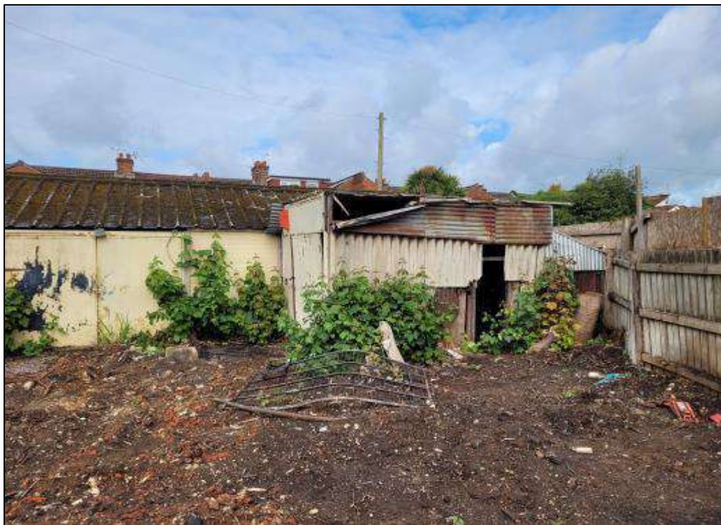
Photograph 2 Showing the small extension on the north-eastern facade
