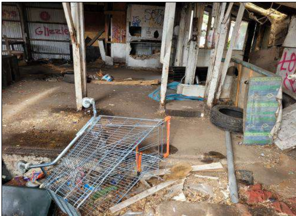
Photograph 3 Showing inside of the building
