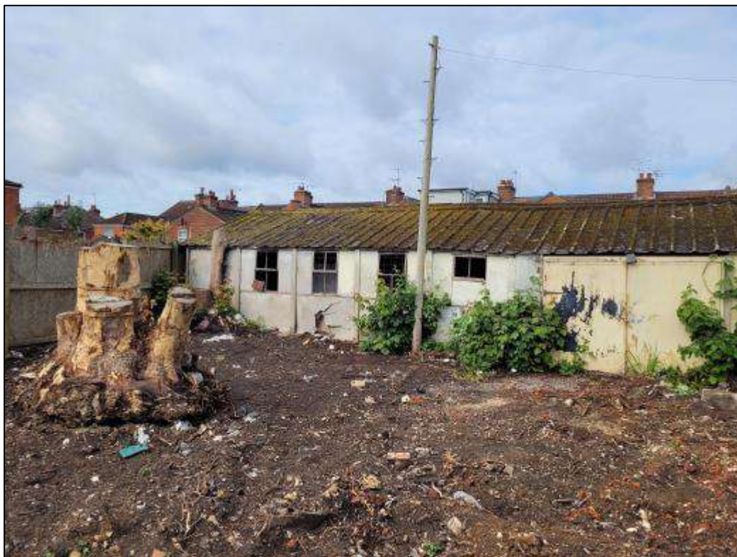
Photograph 1 Showing the former garage building on the western section
