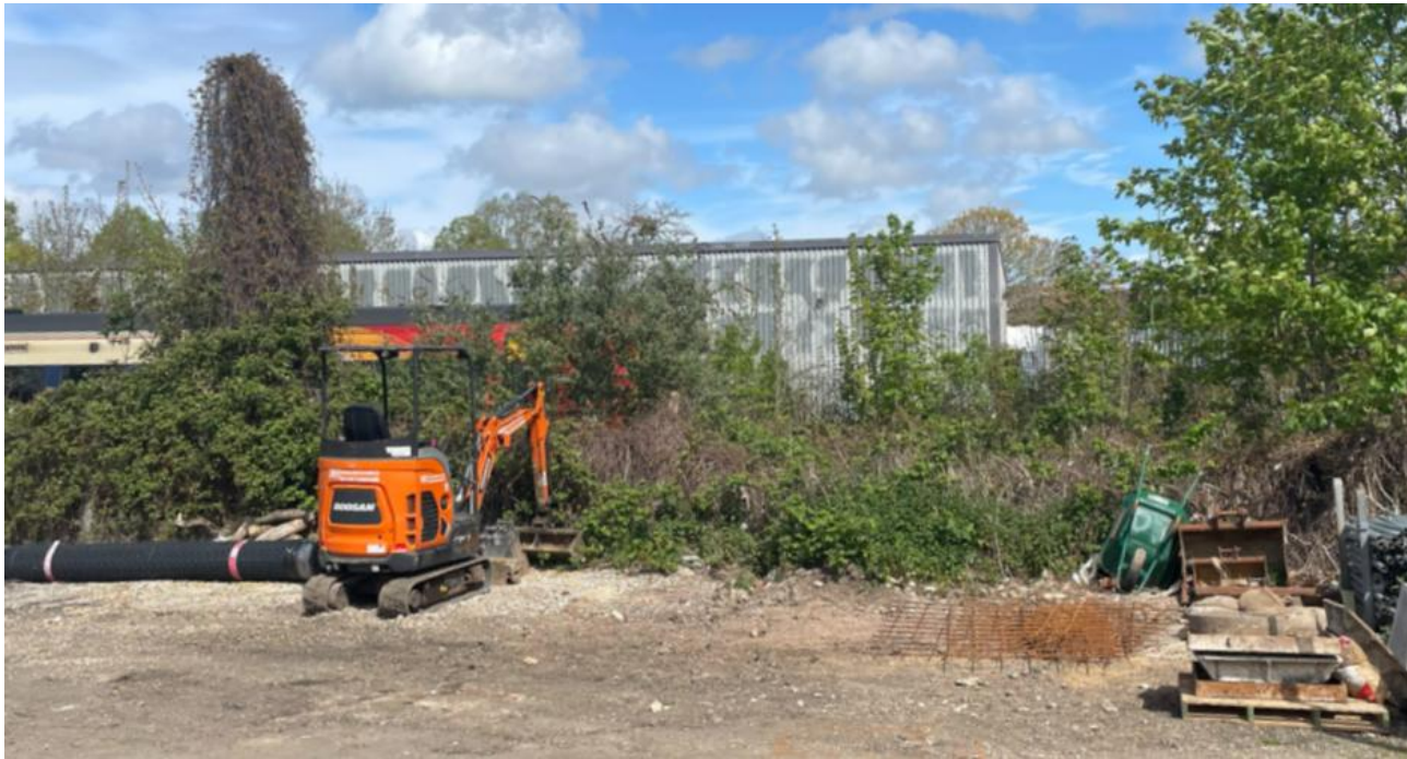
Figure 10 - South Western Railway line adjacent (north) of the site
