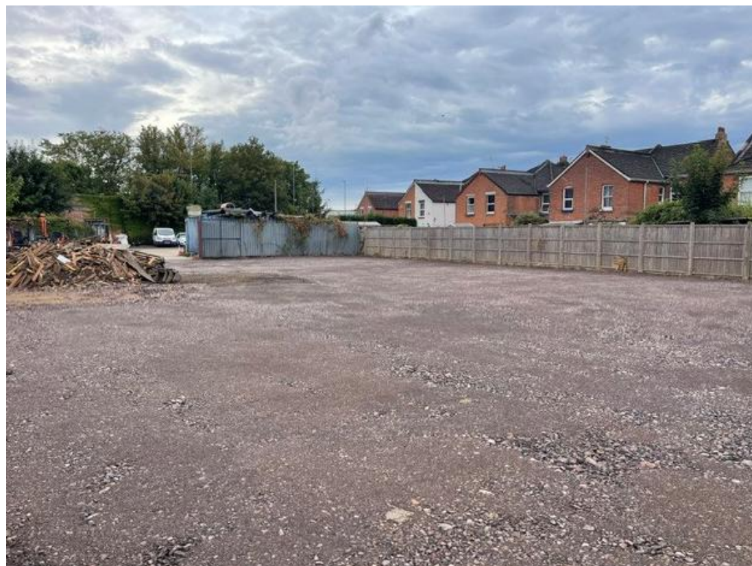
Figure 4 – Site with retrospective limestone hardstanding in place
