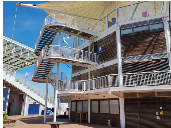
Figure 3.8 Rod Bransgrove Pavilion external walkways
