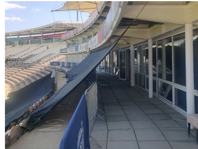
Figure 3.9 Top of Level 00 terrace under level 01 balcony.
