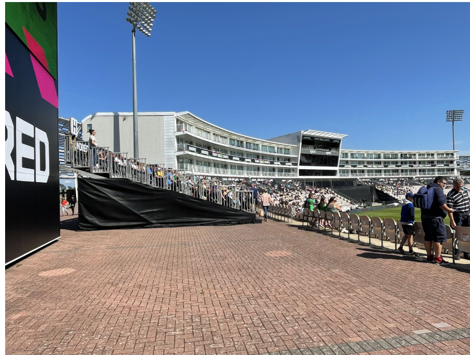
Figure 3.2 View of the external concourse, temporary stands and hotel
