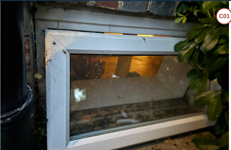
P05 C01 basement window - external view
