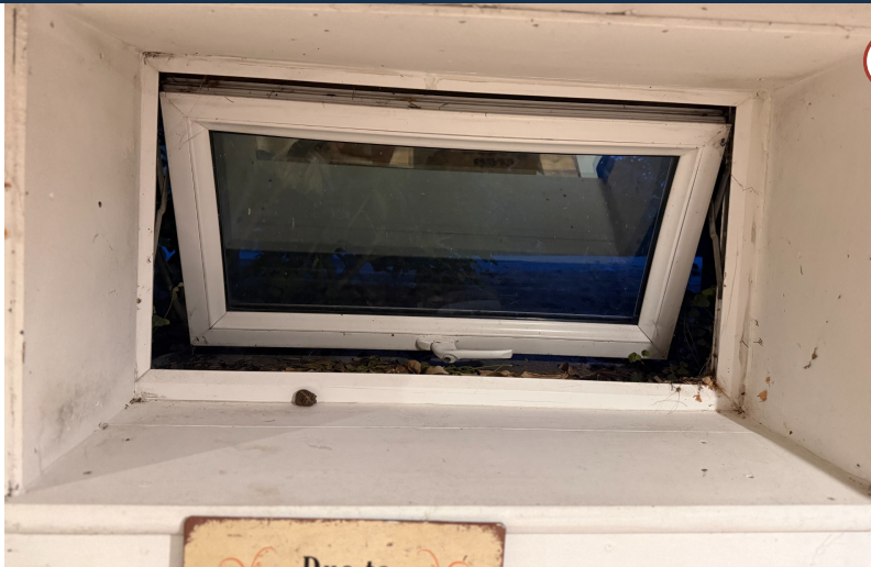
P06 C01 basement window - internal view
