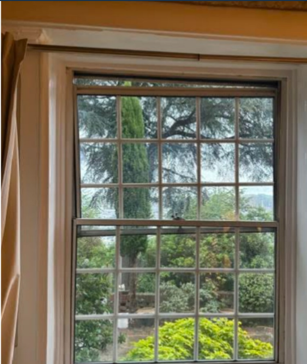
P03 Typical retained surround and later insert
