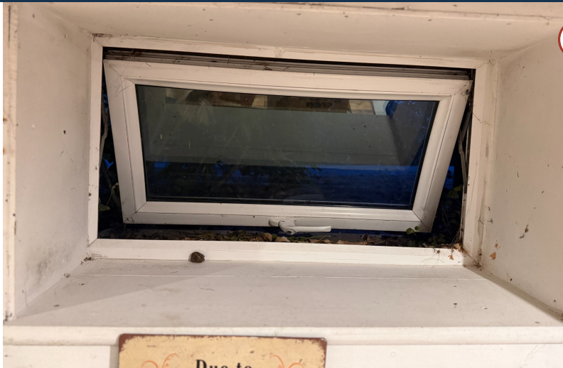
P06 C01 basement window - internal view
