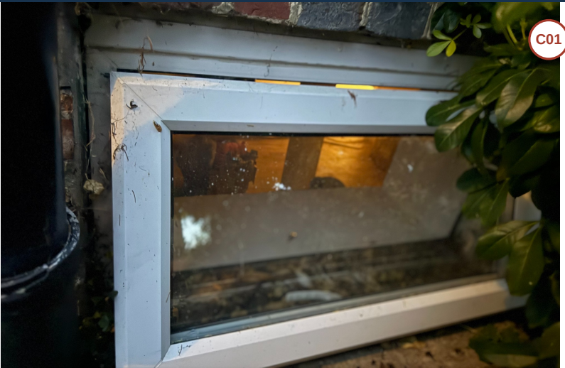
P05 C01 basement window - external view
