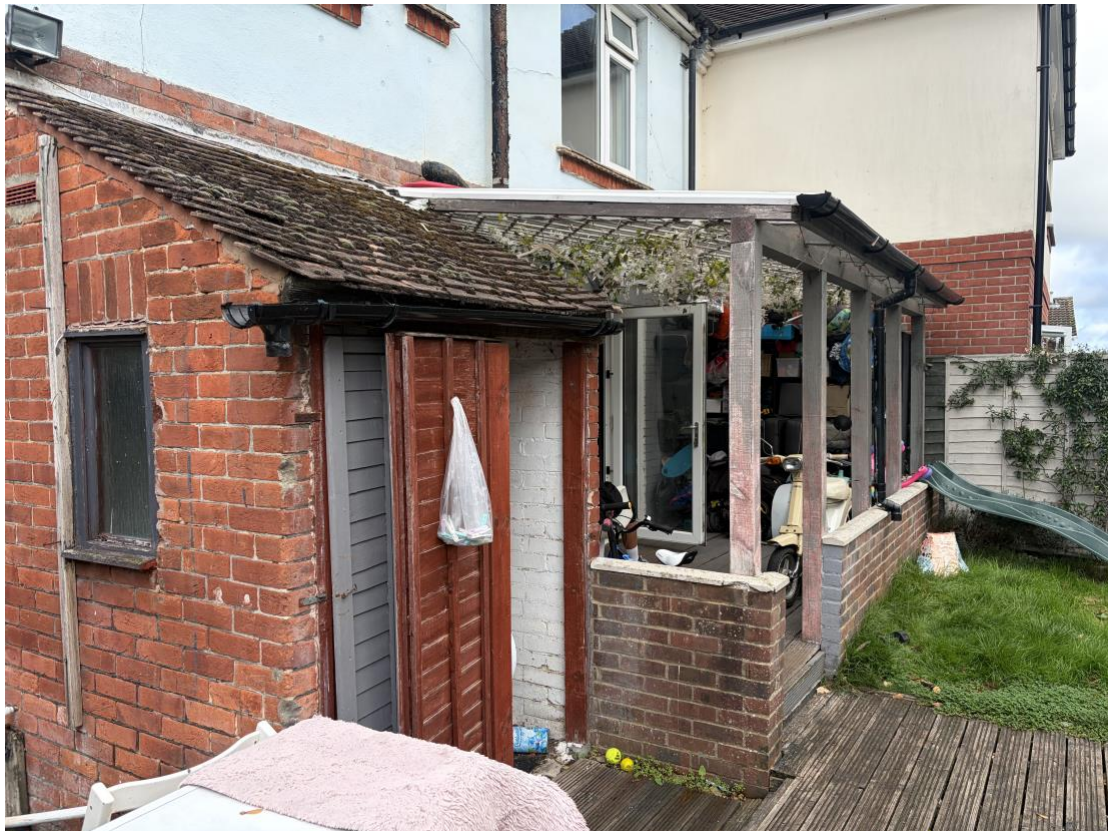
Figure 4. Rear elevation of the 2 Lower New Road property (September, 2026).
