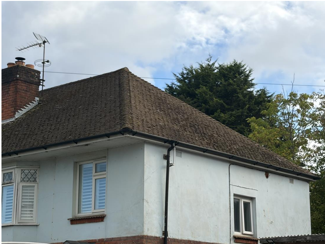
Figure 3. Front elevation of the 2 Lower New Road property (September, 2026).
